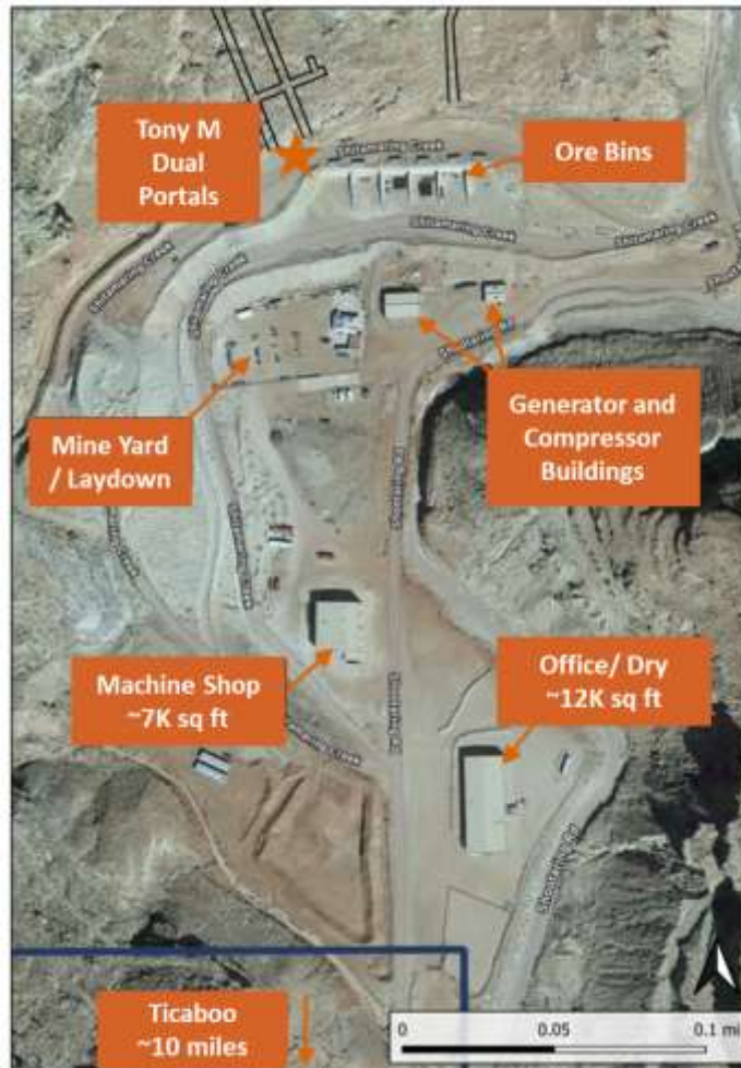
Figure 2 – Image of large-scale surface infrastructure at the Tony M Mine, which includes two parallel declines extending 10,200 ft, a power generation station, fuel storage facility, ore bays, maintenance building, offices, dry facilities and evaporation pond.
